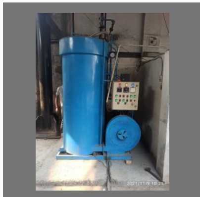
Non lbr Coil Type Steam Boiler
